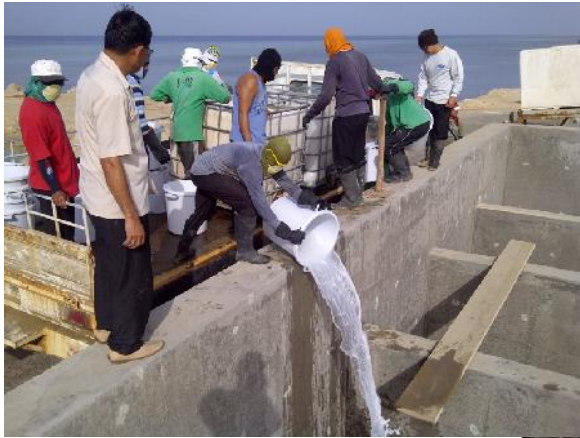
Application of chemicals for disinfection
